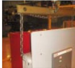
An optional lifting yoke is a simple hook, chain and spreader bar assembly used to lift circuit breakers with an overhead crane or hoist.
